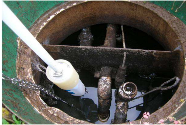
Figure 6: Clarifier C sampling chamber of the CA-5 SBR at the Cromaglass Wastewater manufacturing facility.
