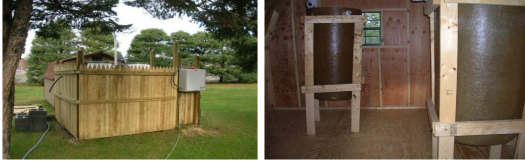
Figure 7A & 7B : The above ground CA-5 at the Williamsport Sanitary Authority on the left. On photograph on the right displays the influent and effluent sampling tees housed inside the shed.
