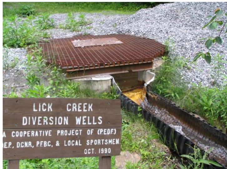
ALDs intercept mine flows and prevent contact with oxygen. They also contain a limestone bed that generates alkalinity transforming the acid water into alkaline water. The water can then be transferred to an aerobic wetland to precipitate out metals before being released into the receiving water body.
