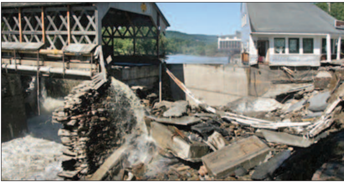
Collapsed bridge/road in Burlington, Vermont after Tropical Storm Lee
