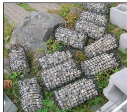
Rock baskets on bank of Susquehanna ready for submersion
