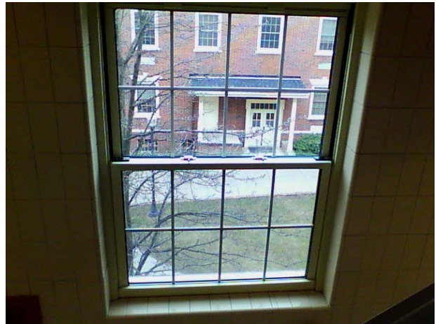
This photo was taken in the stairwell on the second floor and shows an 8.8 degree C air leak around the perimeter.
