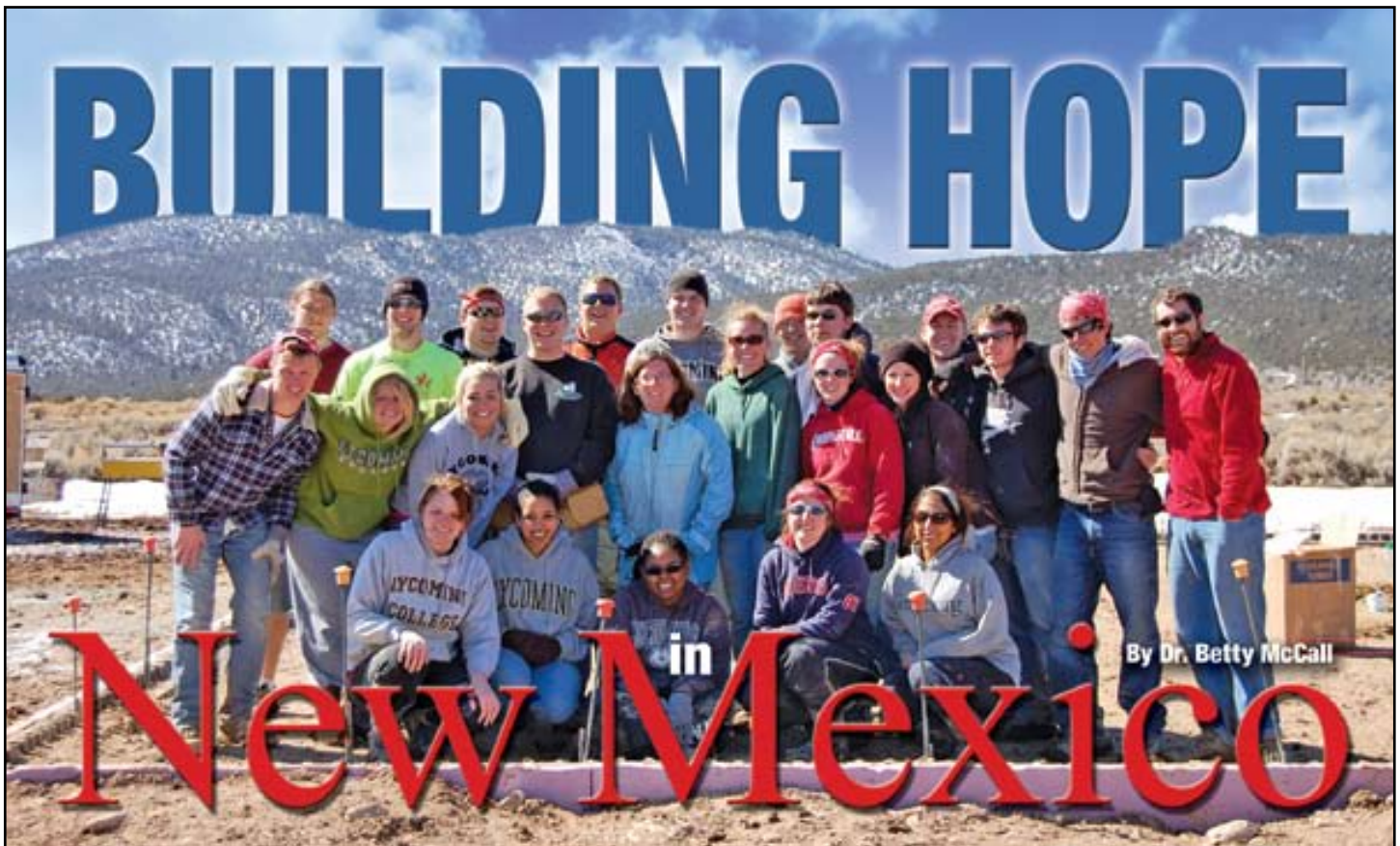
Twenty-four Lycoming students helped lay the foundation for a home in Questa, N.M., as part of the Habitat for Humanity Collegiate Challenge during spring break.
